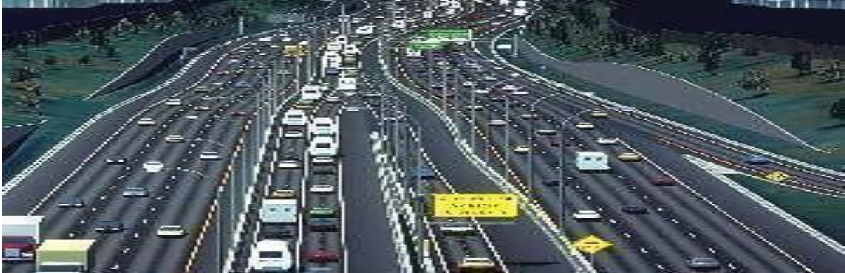
Figure 2.1 –A concept drawing of an Automated Highway System with dedicated lanes in the centre of the highway.
